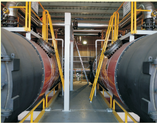
2-Heaters Arrangement (Fire Tubes)
