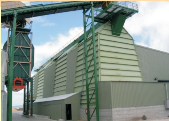
Prefabricated 4 x 400m 3 Quadrant Traverse Silos with Metering Extraction Screws - New Zealand
