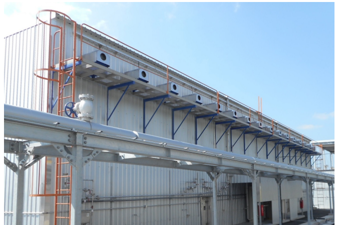
Above: Forklift loaded kilns with fan motors outside for easier servicing.
