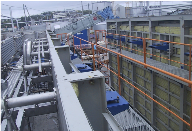
Above: 2 x Rectangular vacuum kilns being installed in Japan.
