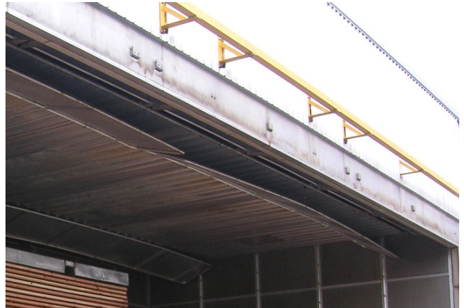
Above: Optional top baffles to help minimize air bypass for better drying results.
