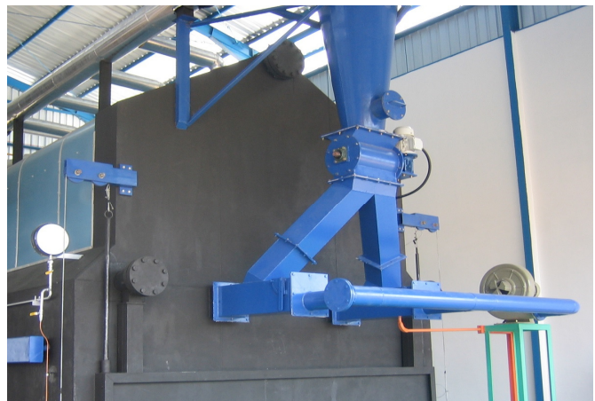
Above: Fuel blow in system. Predominantly for sawdust and shavings.
