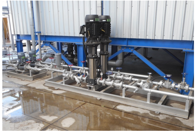
Above: Heat plant feed water pump station.
