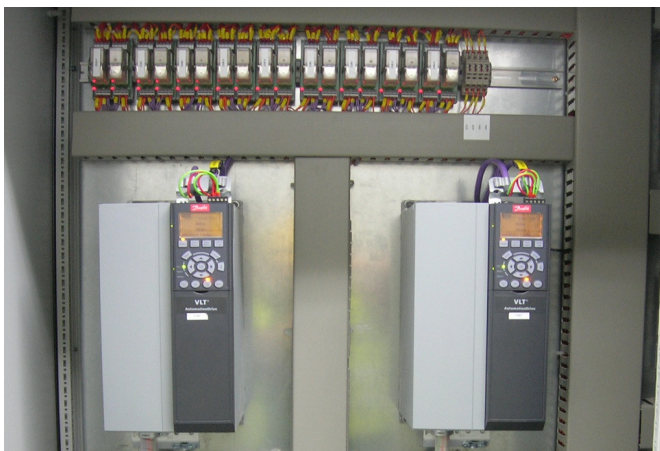
Above: MCC board with variable speed drives shown.
