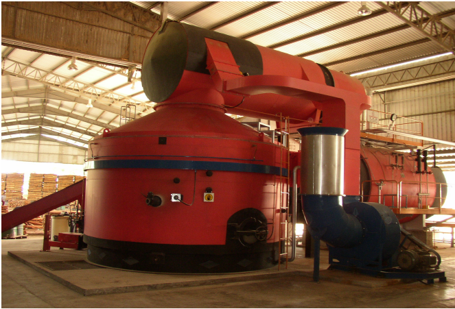
Above: (5MWth, 8000kgs/hr F&A 100°C) Saturated 12barg steam boiler in Malaysia.
