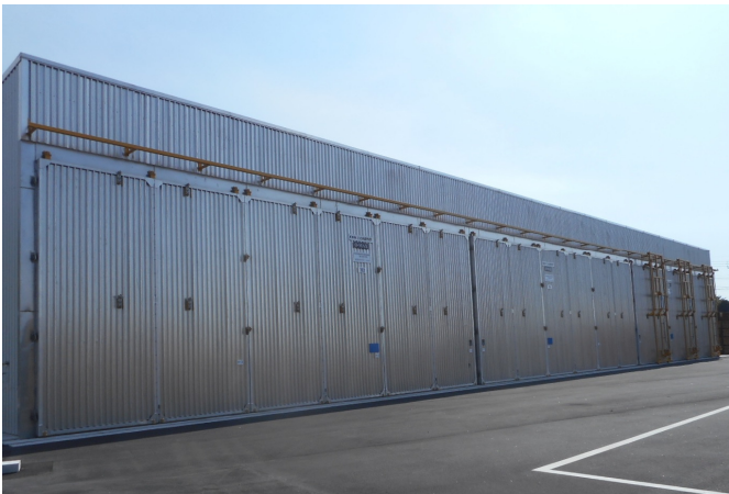
Above: 3 x 100m3 Forklift loaded kilns with fully prefabricated wall panels in Japan.
