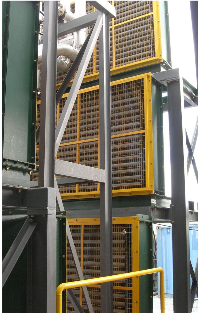
Above: 5MWth heat dump system made out of multiple 1MWth heat dump units.
