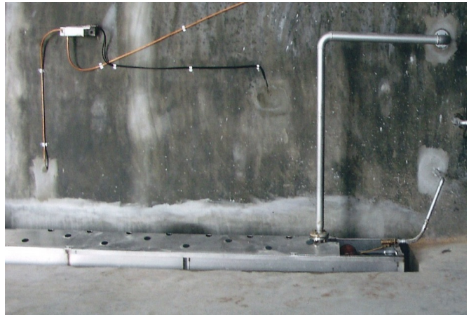
Above: Optional steaming trough system to produce humidification steam at 100degC. Improves drying quality.
