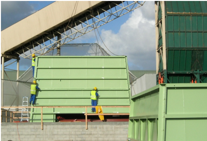
Above: 400m3 Silos being installed layer by layer in New Zealand.
