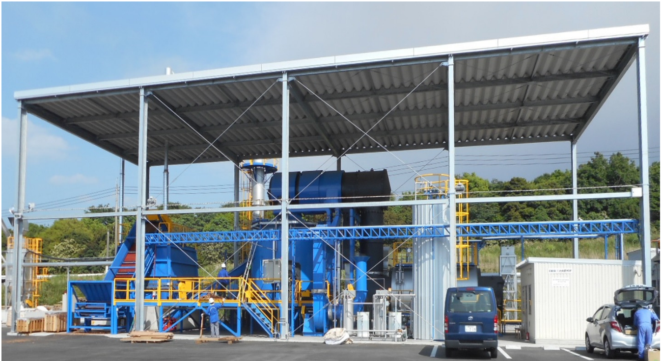
Above: Biomass fired steam boiler plant in Japan with complete fuel handling, civils and ancillaries along with timber drying kilns. This is a complete heat & timber drying plant. See pictures below.
