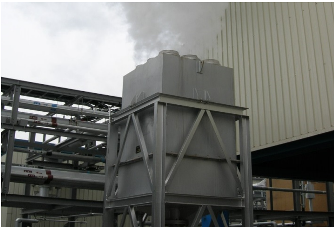
Above: A steam vent silencer for low pressure steam systems.
