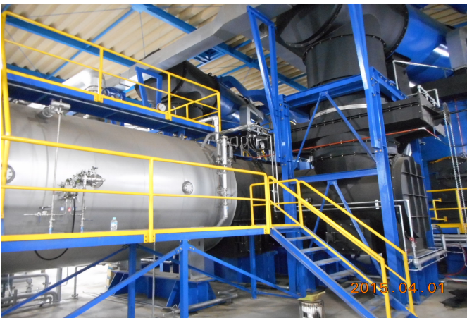
Above: (10MWth, 15,000kgs/hr F&A 100°C) Saturated 10barg steam boiler in Japan. (2 Furnace, 1 Boiler setup)
