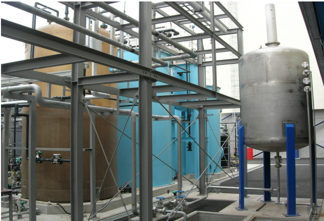
Above: Atmospheric stainless blow down tank.
