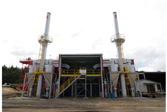
Above: (2 x 4.4MWth) High pressure hot water heat plant in New Zealand.
