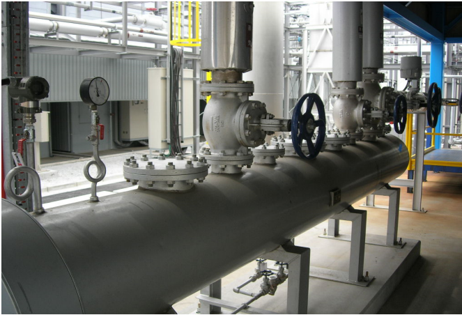
Above: Steam header complete with valves and ancillary instruments.
