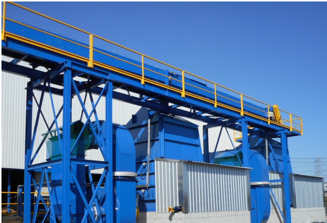
Above: Small fuel daybins and complete fuel infeed system.
