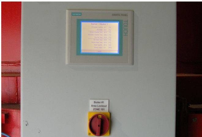
Above: Local board with a HMI touch panel for easier viewing.
