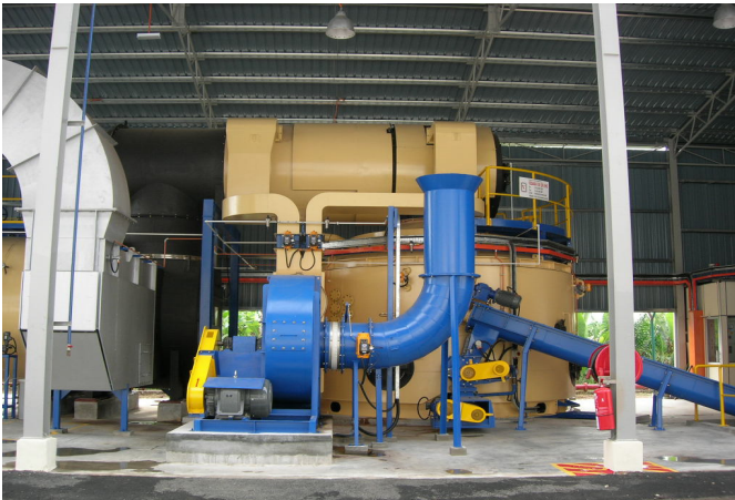
Above: (6.3MWth, 10,000kgs/hr F&A 100°C) Saturated 18barg steam boiler in Malaysia.
