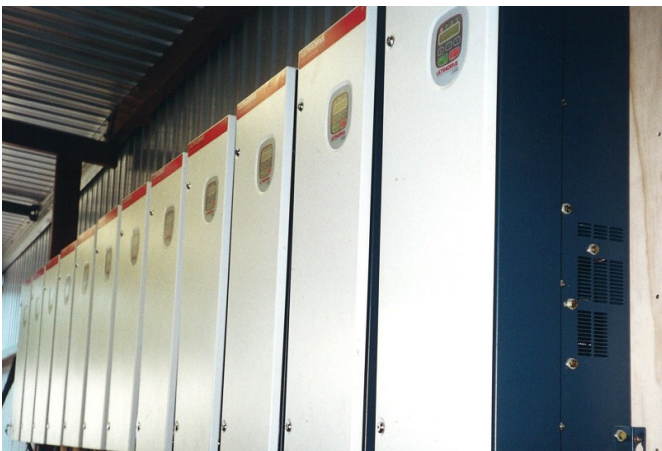
Above: Optional variable speed drives (VSDs) to help save power & enhance drying quality by varying air flow through timber stacks.
