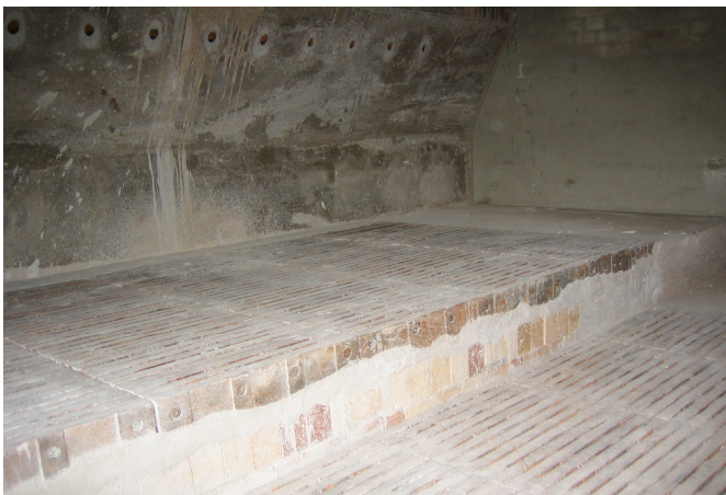
Above: Fixed grates with secondary combustion air nozzles being visible.
